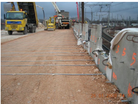
▲ Retaining wall next to the track
