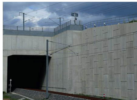
▲ Retaining wall on SEA HSL 3
