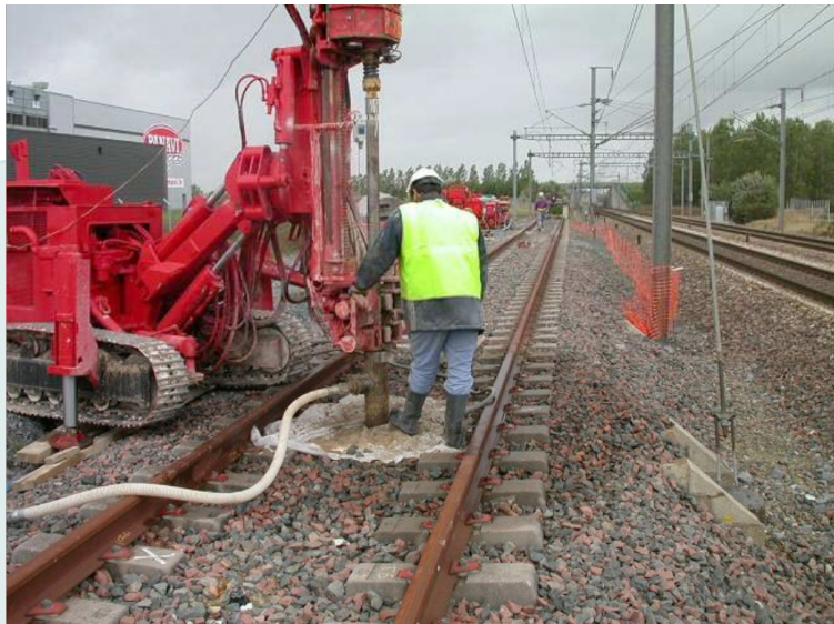
▼ Strengthening a railway subgrade with «Soil Mixing» technology. ▲
