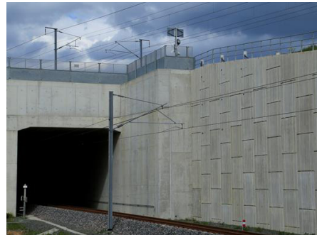
▲ Retaining wall on SEA HSL 3
