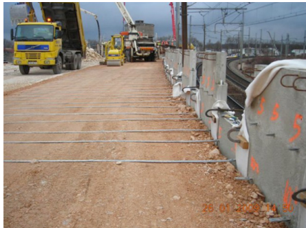
▲ Retaining wall next to the track
