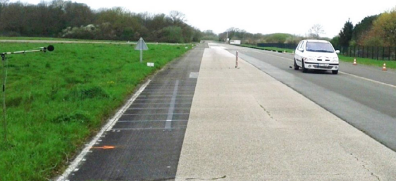
▲ Continuous measurement of embedded system rolling noise.
