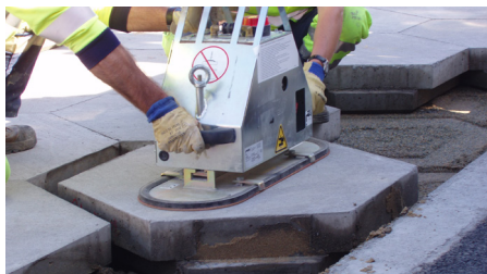
▲ A dismounting-remounting test on Nantes Métropole's dismountable urban pavement demonstrator
