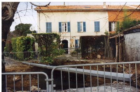
▲ Collapse of a road as a result of the dissolution of gypsum in the subsoil.
