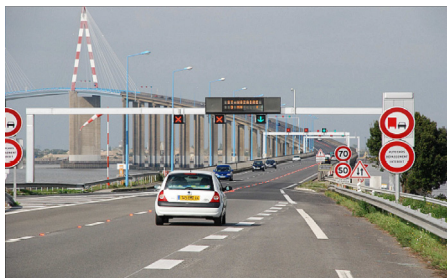
▲ The road communicates dynamically with the user through signage: the central contraflow lane on the St Nazaire – St Brévin bridge.
