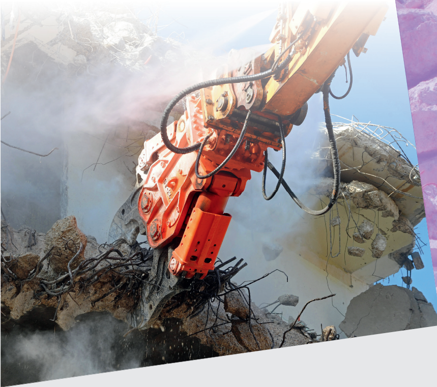
▲ Demolition by pliers
