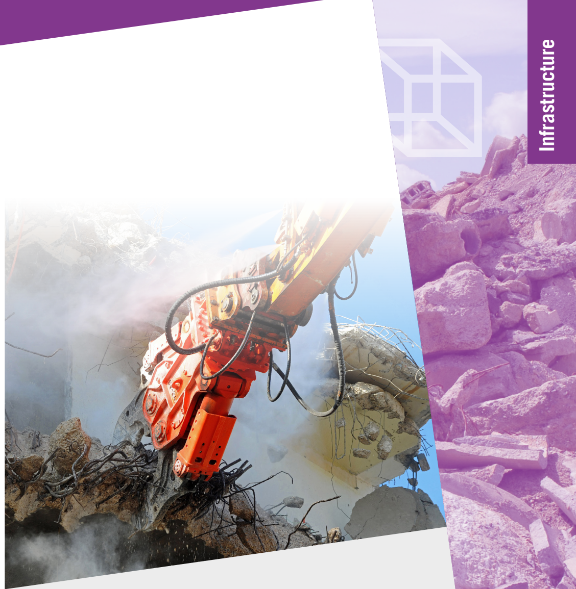
▲ Demolition by pliers
